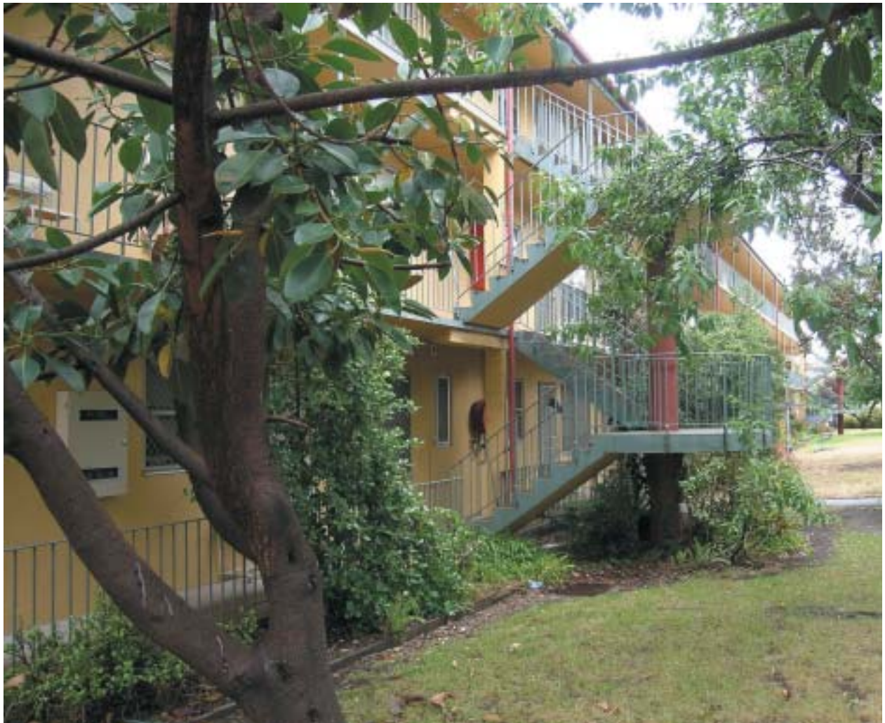
Public governmental housing in Melbourne
