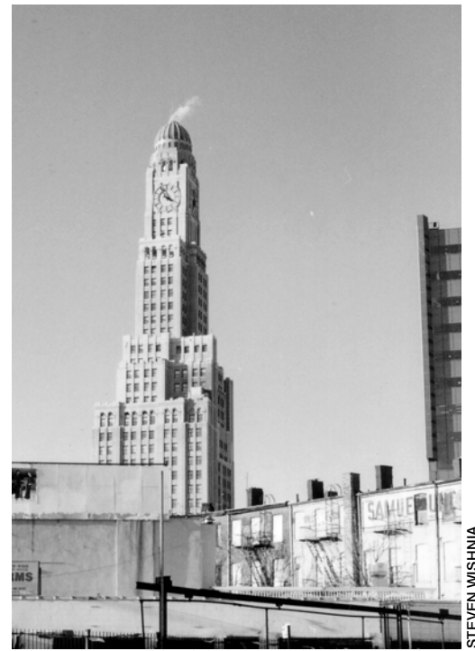
The proposed high-rise would overshadow the landmark Williamsburgh Bank Building.
